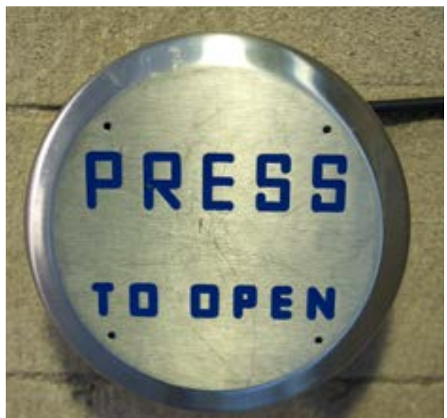
Exit button by the smaller set of toilets
