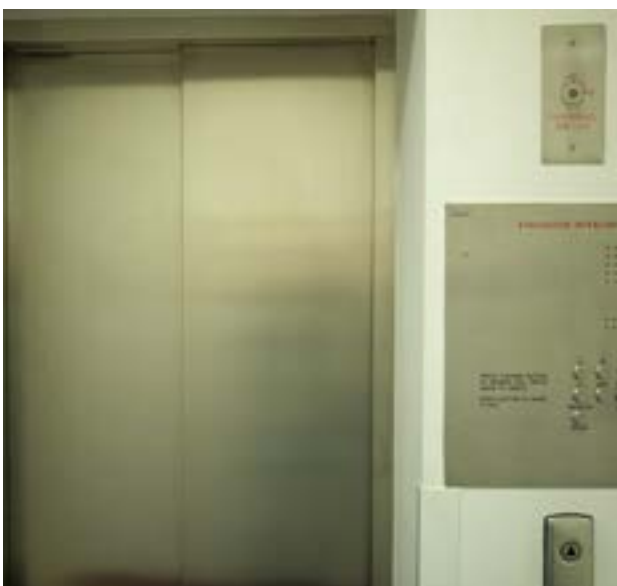
Lower ground floor / accessible entrance
